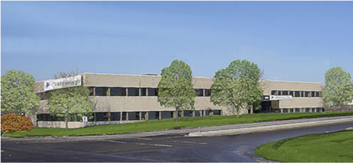
An artist's conception of the Compassion Canada Headquarters, viewing the south-east side of the building.
